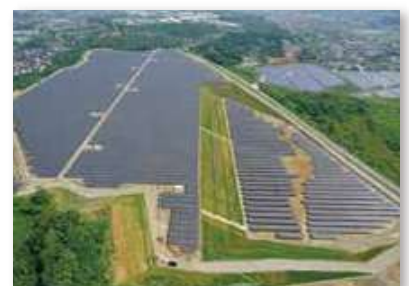
The solar power plant which is operated by Mirai Soden Kami-Mio Corporation (Ownership: Sojitz Corporation – 42%, Sojitz Kyushu Corporation – 18%)
